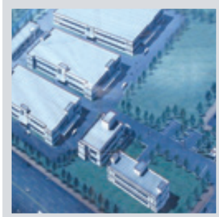
Wuxi Plant (China)
