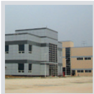
Wuxi Plant (China)
